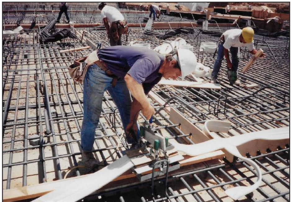
PVC637 (with eyelets: EYPVC637) 6" Ribbed Waterstop 125 ft Head of H 2 O • 50 lft/roll • 1.5 lbs/lft
